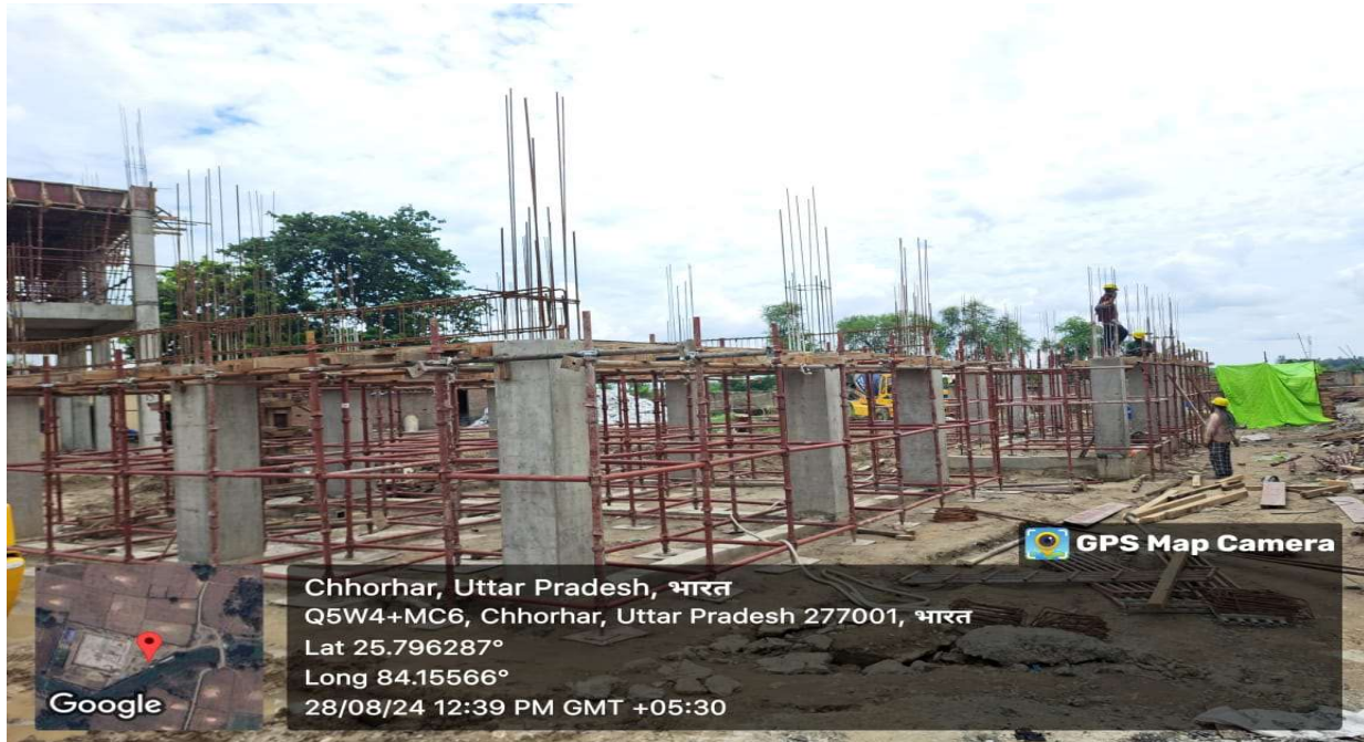
Primary treatment Unit
