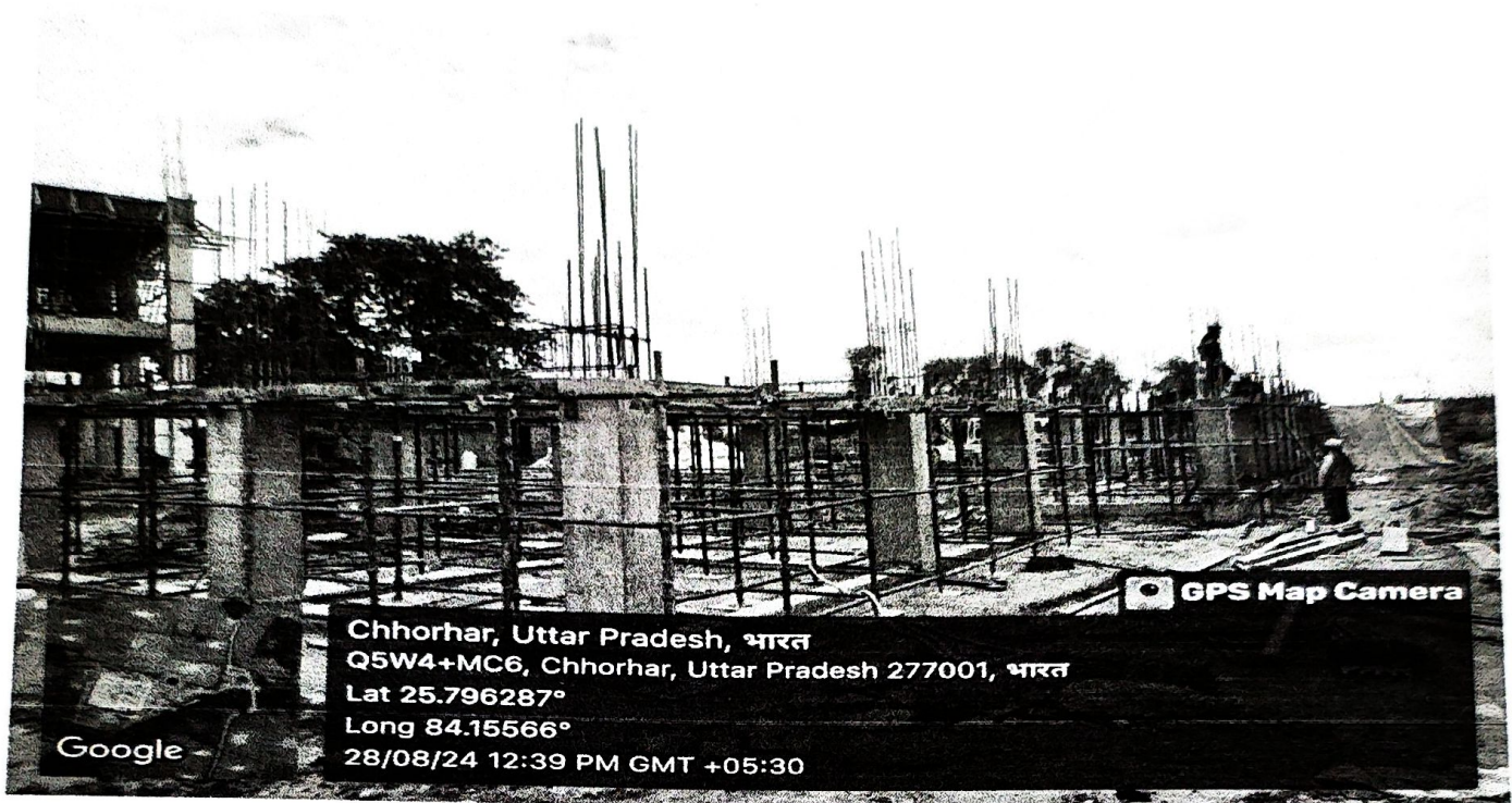
Primary treatment Unit
